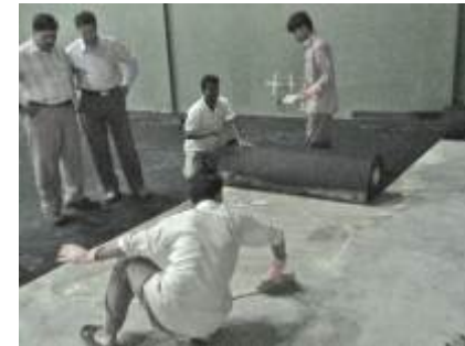
Work under execution - Badminton Court at Club Solaris, Pune ➔
